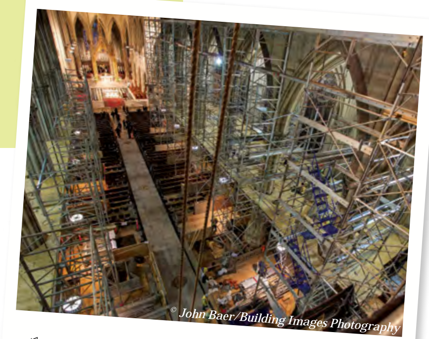
The restoration continues inside with scaffolding reaching the 85ft-high ceilings
