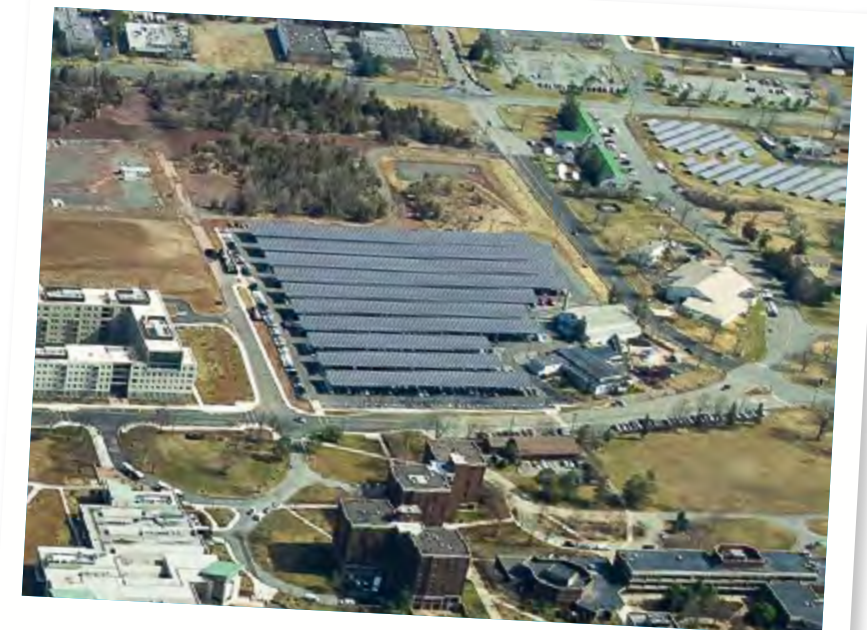
Bird's-eye view of the 31,000 solar panels
