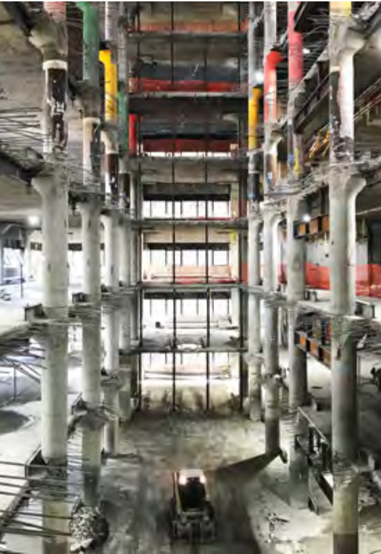
Above ▲ Demolition of existing slabs makes room for a new structural core
