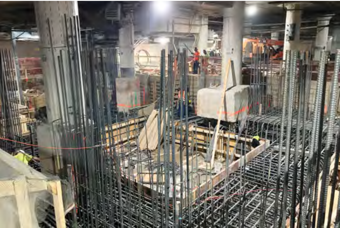
Above ▲ Existing foundations and column footings were strengthened with steel rebar and over 330 yards 3 of concrete in a single pour
