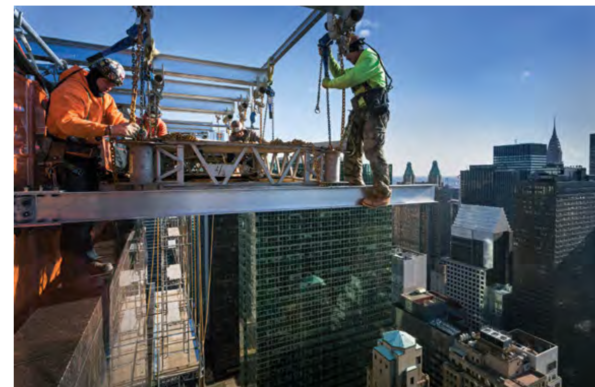
Above ▲ Parts of the scaffold extended up to 6ft over the edge of the building
